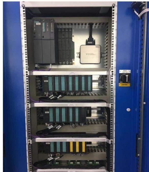
Fig. 3. One of the CPM CPU PLC together with its remote I/O.
